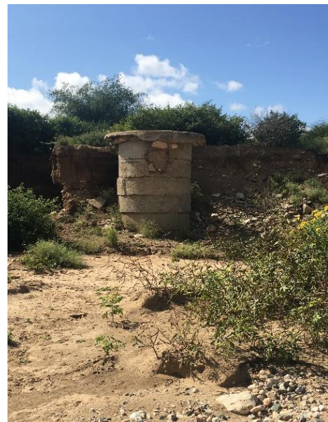
Figure 28a and b. Camud sand dam remains in the left riverbank and exposed concrete-ring well next to the collapsed dam. Source: Lopez-Rey (2019)
