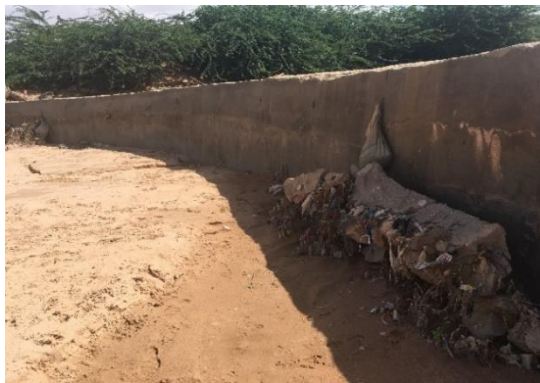
Figure 10a and 10b. Fully eroded gabion and exposed steel bars on the crest of Aw Barkhadle sand dam. Source: Lopez-Rey (2019)
