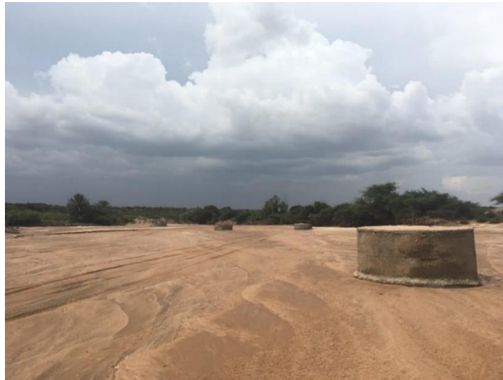
Figure 20. Masonry communal and private wells in the throwback of the oldest sand dam in Hulusuq built in 2000. Source: Lopez-Rey (2019)
