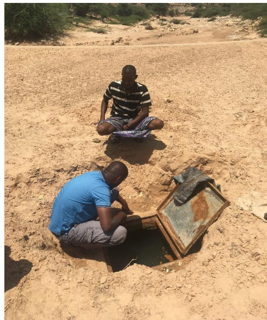
Figure 15. View of the new well 10m upstream of Diinqal sand dam. Source: Lopez-Rey (2019)
