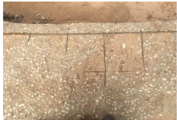
Figure 10a and 10b. Fully eroded gabion and exposed steel bars on the crest of Aw Barkhadle sand dam. Source: Lopez-Rey (2019)
