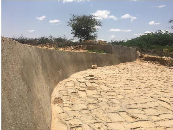
Figure 14. View of the left wing wall and riprap in Diinqal dam Source: Lopez-Rey (2019)
