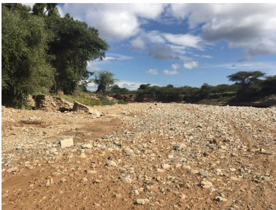
Figure 28a and b. Camud sand dam remains in the left riverbank and exposed concrete-ring well next to the collapsed dam. Source: Lopez-Rey (2019)
