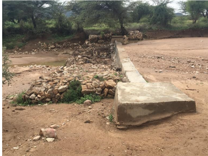
Figure 25. View of insufficiently extended wing wall on the left bank and partially washed-away gabions in Carracad dam. Source: Lopez-Rey (2019)
