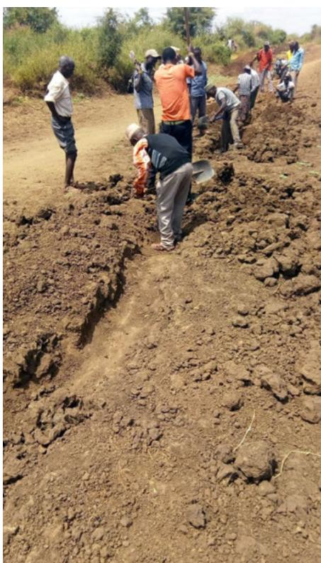
Figure 5: Ramole community in Marsabit County working on a trench for water piping from a borehole to their village as part of their Disaster Risk Reduction (DRR) plan in 2020. Photo: Rob Galgallo
