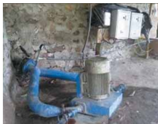
Fig Peltric set unit for electricity generation at Sirise, Udayapur district, 2010. Photo: Shiva Basnet
