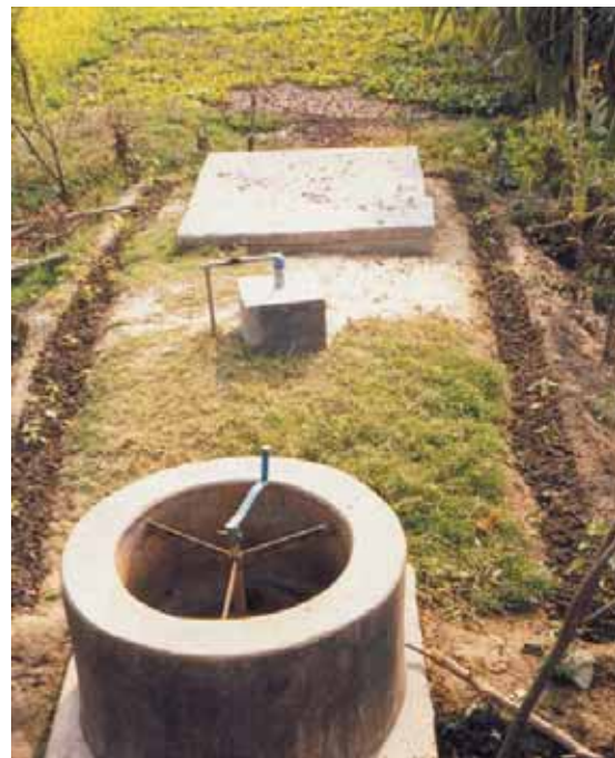
Fig Bio Gas Unit.
