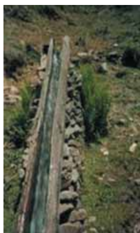
Fig Traditional penstock made of wood
