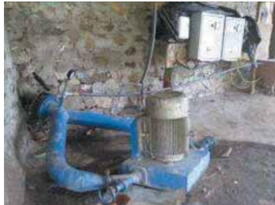
Peltric set unit for electricity generation at Sirise, Udayapur district, 2010. Photo: Shiva Basnet
