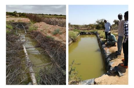
Figure 9 - Water basins lined with plastic sheet with (left) or without (right) cover (to reduce evaporation). These structures are located beside tree orchards or gardens and provide water for irrigation during dry spells or the longer dry season. Photo taken by Cecilia Benda (2014).
