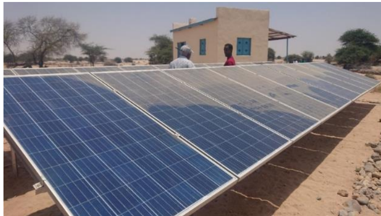
Figure 20: A solar array in Somaliland that has only been partially cleaned and so will not be operating at full capacity
