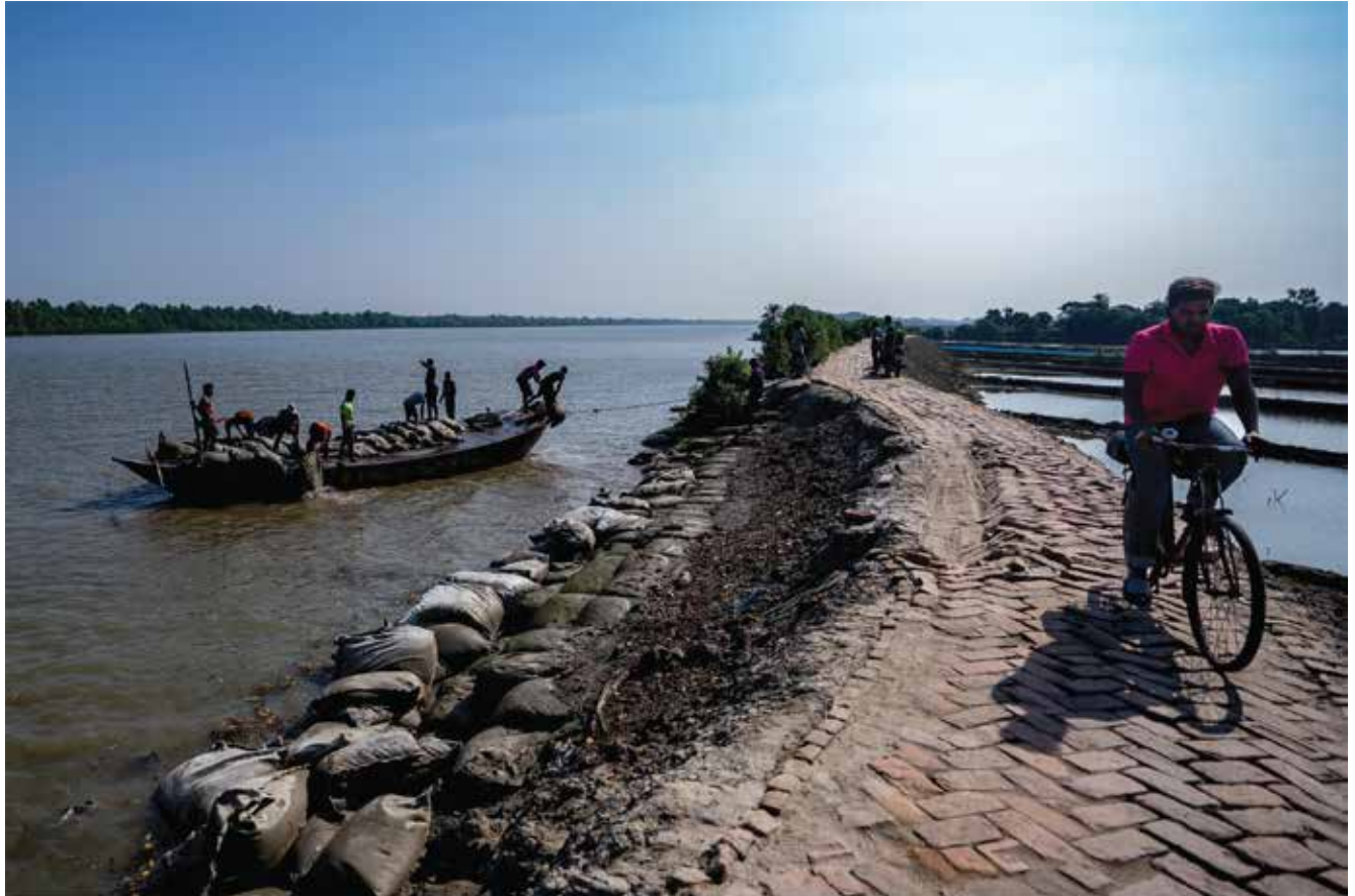
A brick road constructed in the embankment of the river Rai in North Bedkashi, Koyra. Each year the road is damaged and slides thinner, flooding the cultivable land with salty sea water on the other side.
