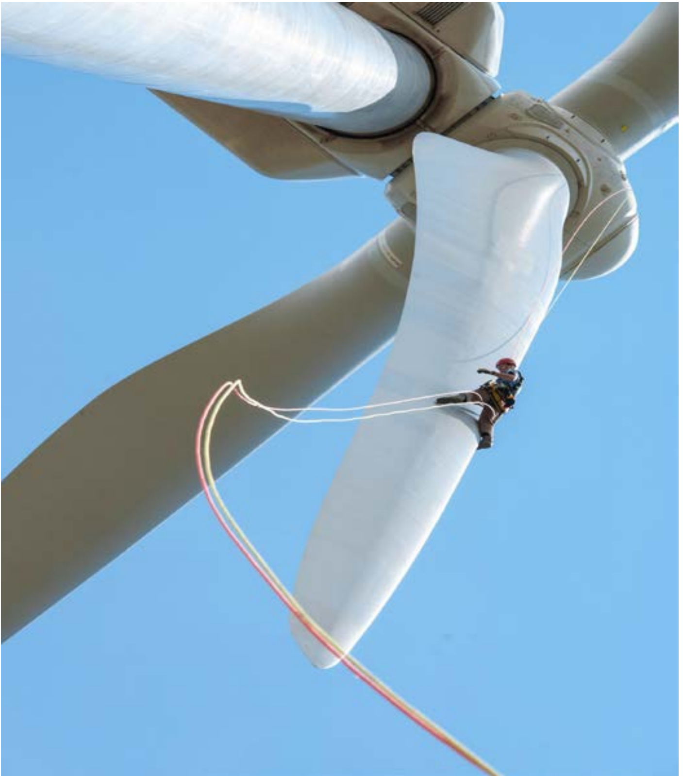
Photo: Inspecting a wind turbine. Photo credit Dennis Schroeder / NREL GPA Photo Archive (Creative commons)
