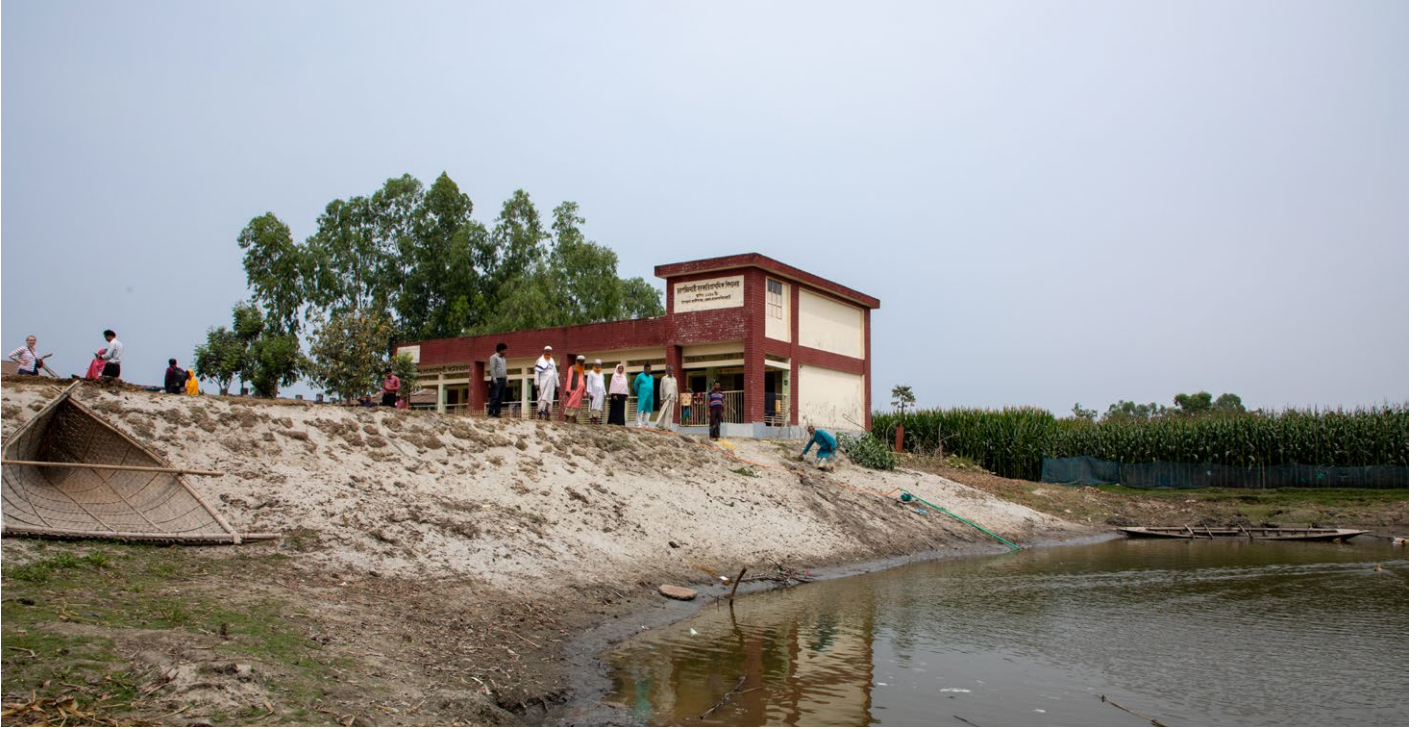
In Daunbni, Rangpur, the 17 member committee meet once a month to represent their 1600 households. The group works with Concern through local partners. They have worked on reconstructing embankments for flood resilience. They have also built pathways to make movement easier during floods. Photo: Gavin Douglas/ Concern Worldwide
