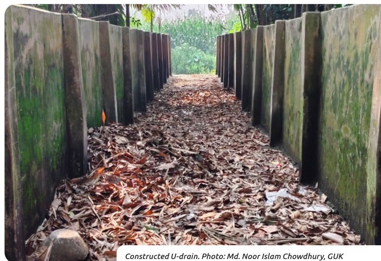
Constructed U-drain. Photo: Md. Noor Islam Chowdhury, GUK
