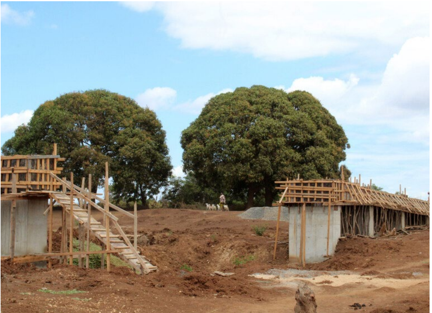
A new bridge under construction at Handaraku, as a result of community-led advocacy efforts. Photo: Charlotte Woellwarth/Concern Worldwide.
