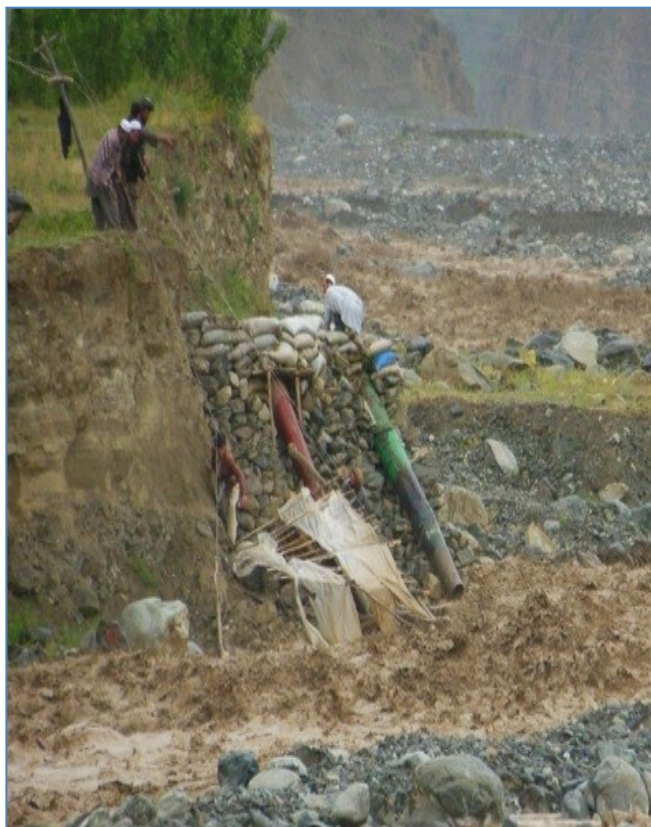
In Badakhshan, Afghanistan, community members scramble to salvage a small hydroelectric power plant from being destroyed due to channel erosion.
