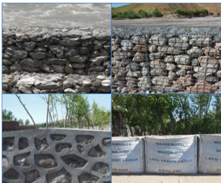
Clockwise from top left: welded mesh gabions, Hesco cells, masonry walling, Big Bag System
