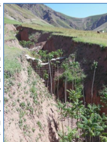
Using bioengineering to reclaim a gully
