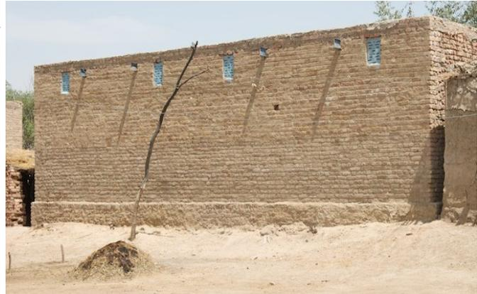
*A reconstructed house in Pakistan: constructed on a plinth, the bottom third is waterproof, the top two thirds are mud brick. (Photo Dom Hunt 2012)*
