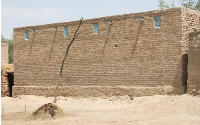
**A reconstructed house in Pakistan: constructed on a plinth, the bottom third is waterproof, the top two thirds are mud brick. (Photo Dom Hunt 2012)**
