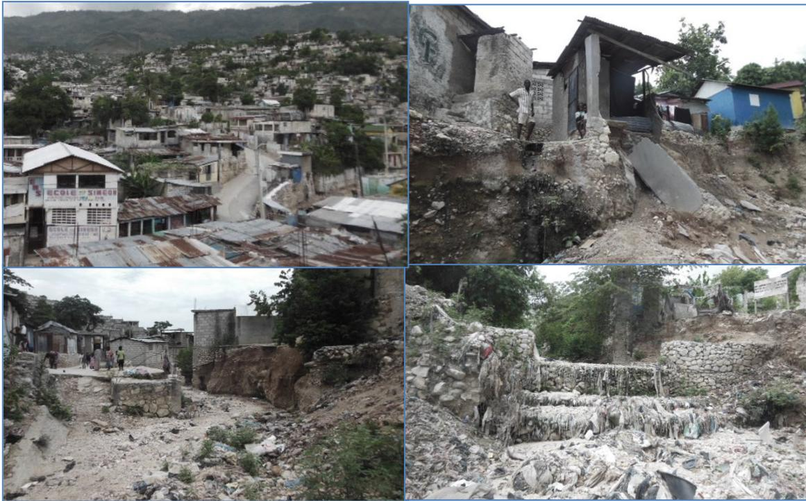
*A number of houses near the gully in the Grand Ravine have been destroyed or are threatened by erosion. Concern constructed two check dams to reduce gully erosion, however they are showing signs of wear (bottom right photo).*
