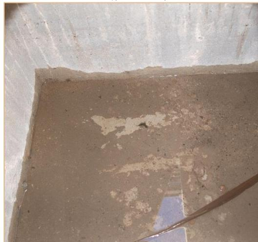
10) Interior of tank – showing pipes for water no method for preventing buildup of sediment from entering tap, Mastheley, Malal Mara
