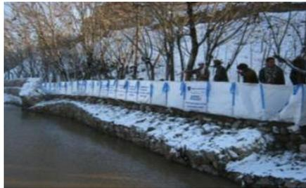
Above: Flood defence made from geotextile cells filled with earth. Photo by Tom Dobbin 2012.
